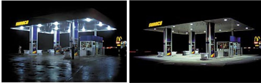
The above photographs illustrate the impact of glare on a lighting installation. The left photo has high-glare, non-recessed fixtures under the canopy. Note how bright the lights themselves are and how dark the pump area is. The right photo shows the same gas station canopy with full-cutoff, recessed fixtures. Note how the light is directed effectively toward the gas pumps. Images from http://www.skvandtelescope.com
